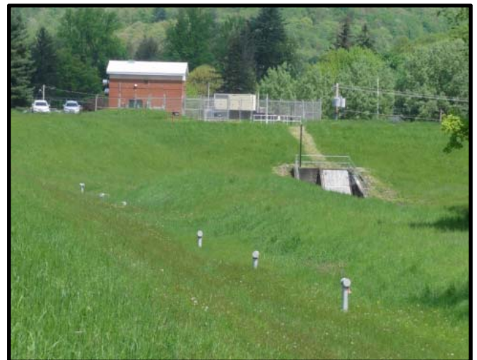
View of Portville Flood Control Project with wells to be replaced along the levee's edge.
